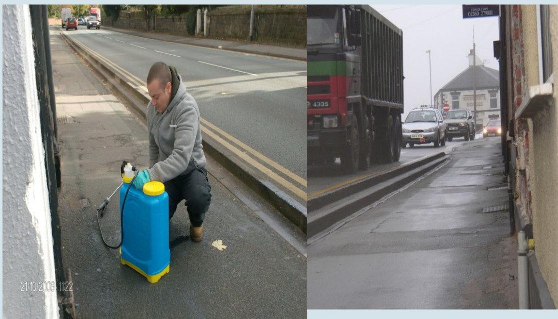
Photo: application of Photo-catalytic paint (left) and the area sprayed (Right) in West Road, Congleton
